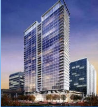
WallStreet Tower as it was originally intended. New architectural drawings will be made.
